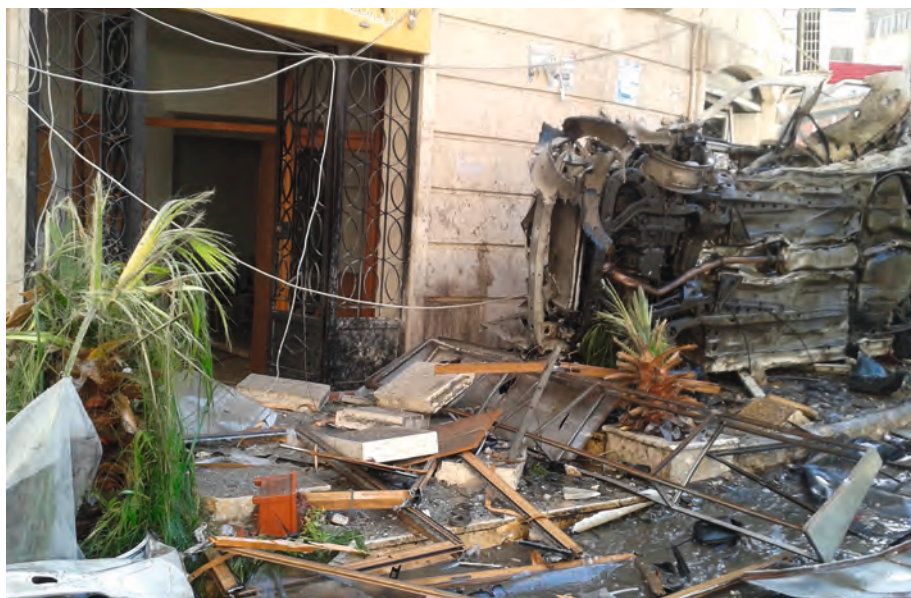
Random rocket falling brought damage to a church in Aleppo
